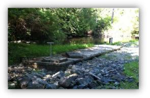
located just upstream of the dam, conveys water through a course screen before entering a 250 mm diameter intake.
